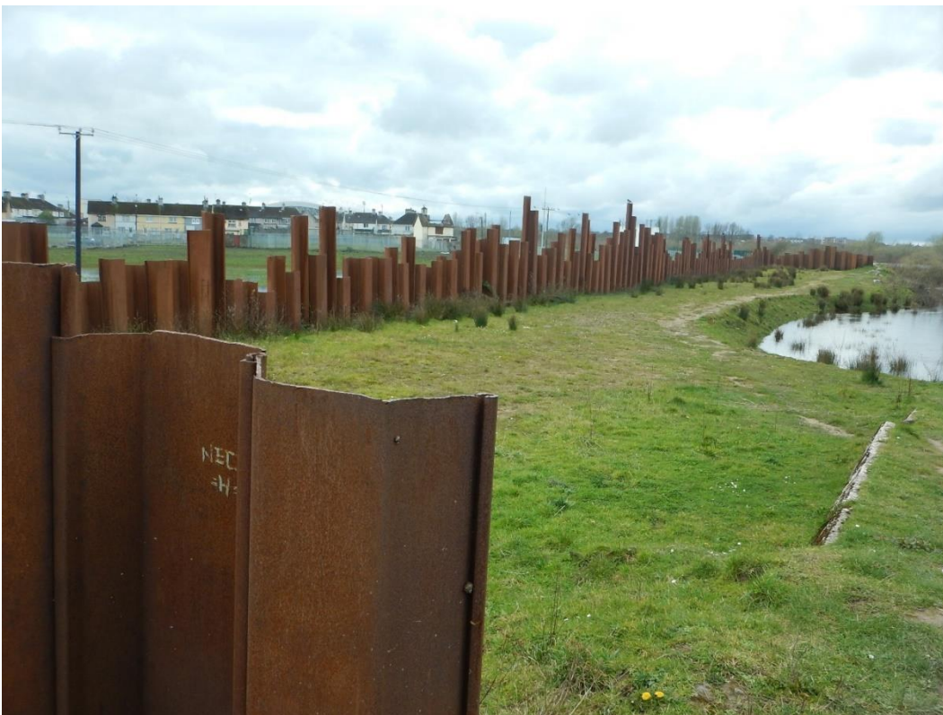
Plate 8-13: Sheet piling and earthen pathway
